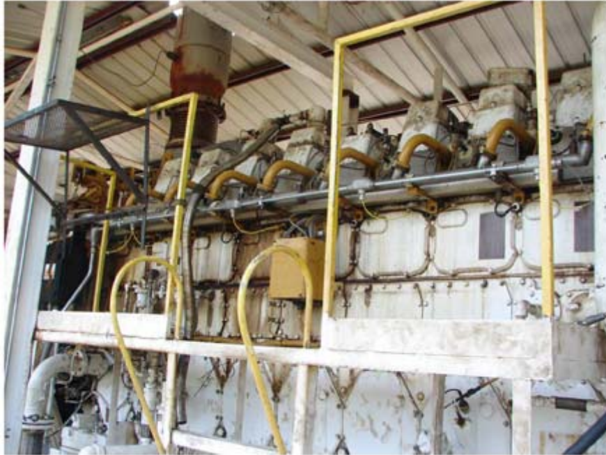
Figure 8-1 - Caterpillar 3608 Engine Under Test
